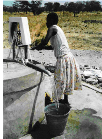
rope pump installed on a hand dug well
