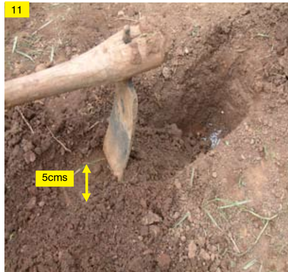
Backfilling Basins: Backfill basins with hoe blade leaving only small hollow about 5cms deep.
