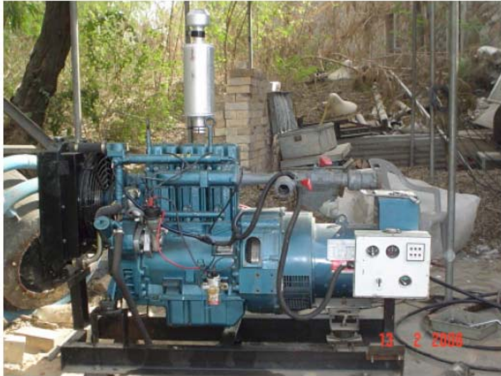
A view of the modified diesel engine with spark ignition system
