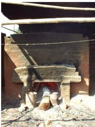
The Traditional Portuguese style oven is different. The bread is baked using conductive heat that is transferred from the combustion chamber into clay bricks and then directly into the bread itself. Higher temperatures are needed in this style of oven (approx 300 Celsius). **The traditional oven is extremely inefficient, relatively expensive to build and is not very durable.**
