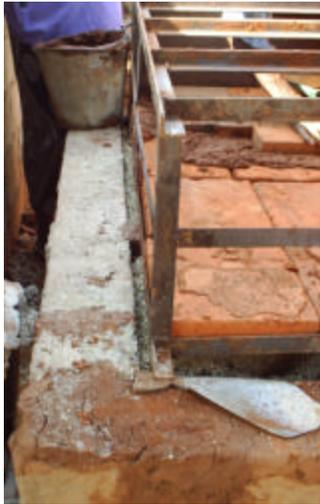
... and then around the **bottom corner of the baking compartment of the oven**. A 3 cm gap is left between the bottom corner of the metal frame and the loose vermiculite insulation underneath. A 2.5 cm gap is left between the oven body and the bottom side edge of the T-bar baking compartment.
