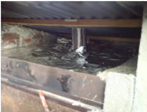
A layer of aluminum foil is placed on top of the vermiculite. More vermiculite is used to hold the aluminum foil in place
