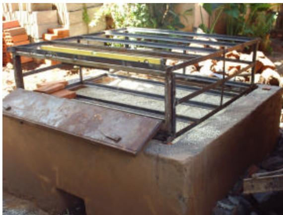
In March 2004, a new bread oven was designed that utilized a 5 mm T-Bar frame to directly support the clay baking tiles instead of the 2mm mild steel sheet metal baking compartment. The use of any metal in the baking compartment is an interim measure to assess if the general concept is acceptable to the bakers. The fourth prototype will not have an angle iron frame on the bottom of the baking compartment and will instead be supported entirely by clay bricks.
