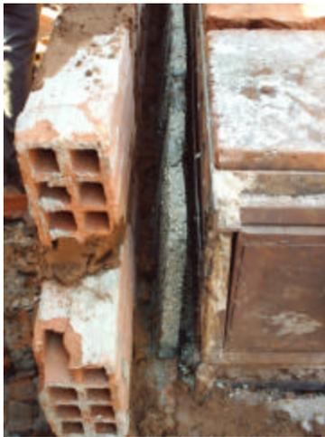
The hot flue gases then travel through the 2.5 cm gap between the T-bar baking compartment and the thin cement vermiculite bricks. The gap between the cement vermiculite bricks and the outer structural bricks will be filled with loose vermiculite. Loose vermiculite is a much better insulator than vermiculite mixed with cement. This is why we use only a thin cement vermiculite tile, thus leaving more room for the loose vermiculite.
