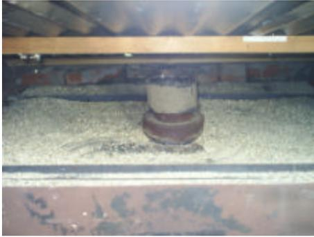
The top of the baking compartment (and in between the supporting outer bricks and the thin cement vermiculite bricks) is insulated with one bag of vermiculite.
