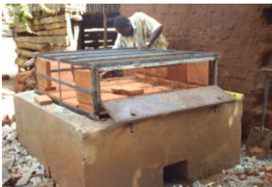
The heat flow was also modified in the second prototype. In the original oven the heat flowed only around the **outside** of the baking compartment. The new
