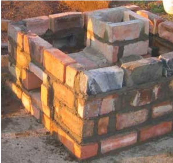
LOWER SECTION SHOWING FUEL FEED HOLE
