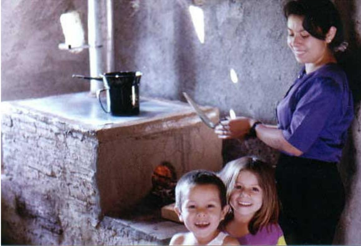
**Is similar to the Estufa Justa de dos hornillas with the exception that there are no holes in the metal cooking surface (plancha). This modification is to accommodate the cultural desire for soot free pots. Unfortunately, the absence of openings in the plancha means a decrease in its efficiency. Both versions of the Estufa Justa can be constructed with an oven with only a slight increase in cost. This oven can easily attain 300 degrees Fahrenheit.**
