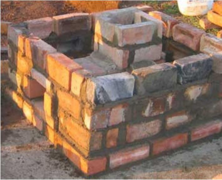
LOWER SECTION SHOWING FUEL FEED HOLE
