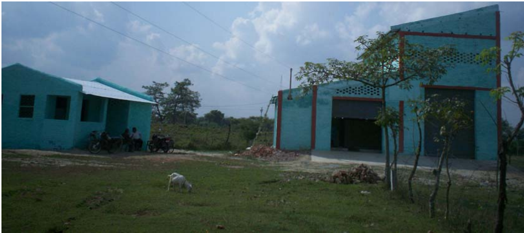
Power plant building with guest hose in Gaiyari
